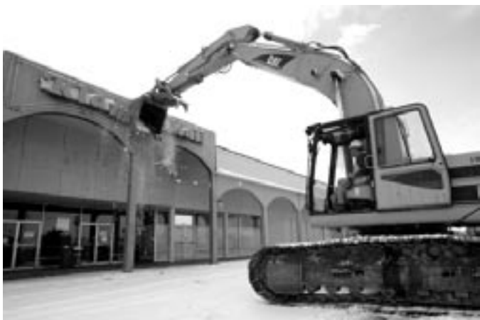
Klamath Mall Demolition, Photo by Gary Thain
